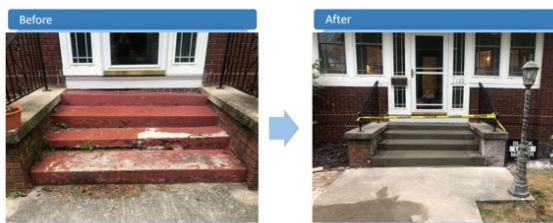
Replaced four cement porch steps. 2021 Block Grant Challenge program participant.
